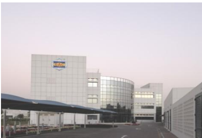
GAC headquarters in Dubai.
