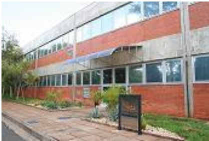
Eldorado office building in São Paulo, Brazil
